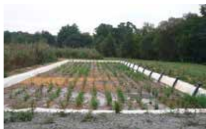
Extension station épuration
